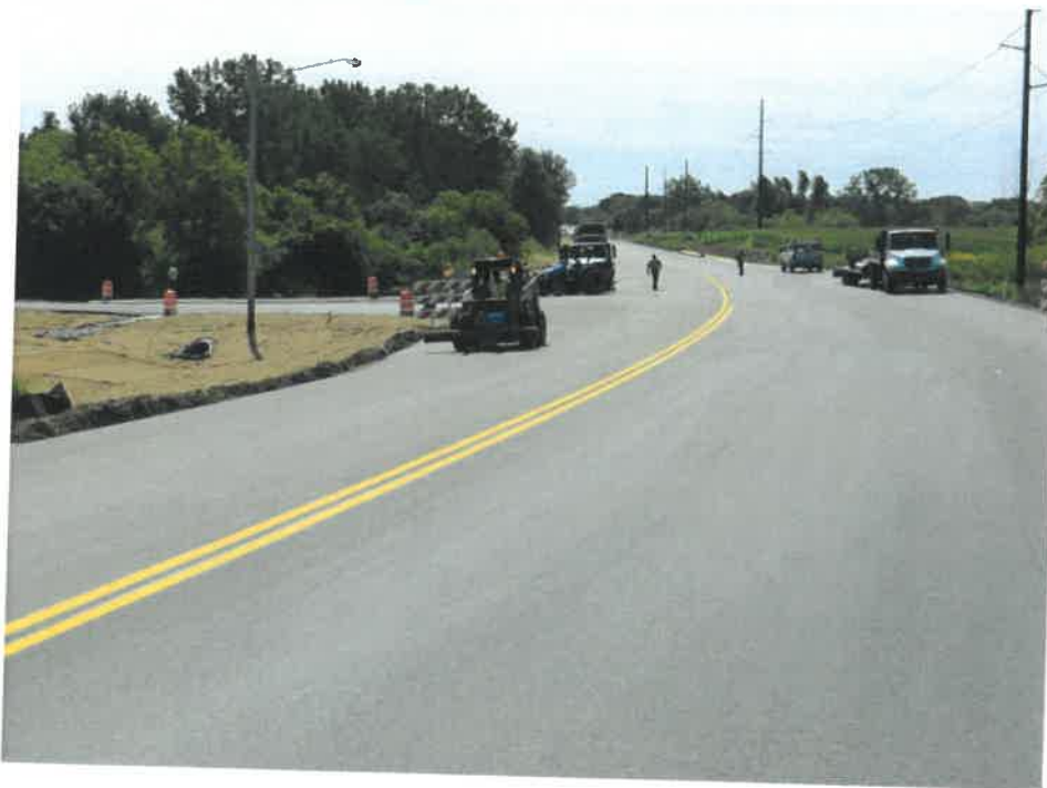
Pavement markings & landscape restoration on new HMA surface
