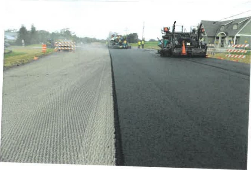
Paving HMA surface
