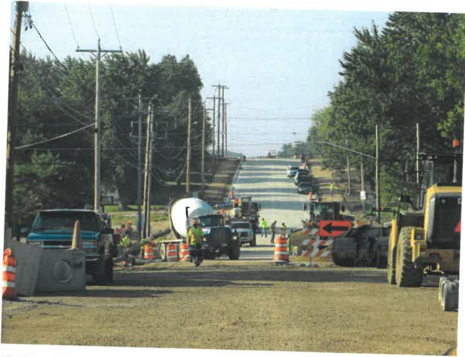
Finished concrete pavement, concrete hand pours, sidewalks prepared for concrete
